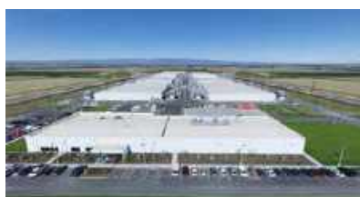
Datacenter Quincy, WA
